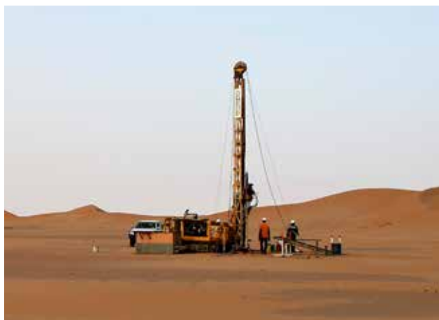
Validation diamond drilling at Hippolyte.
