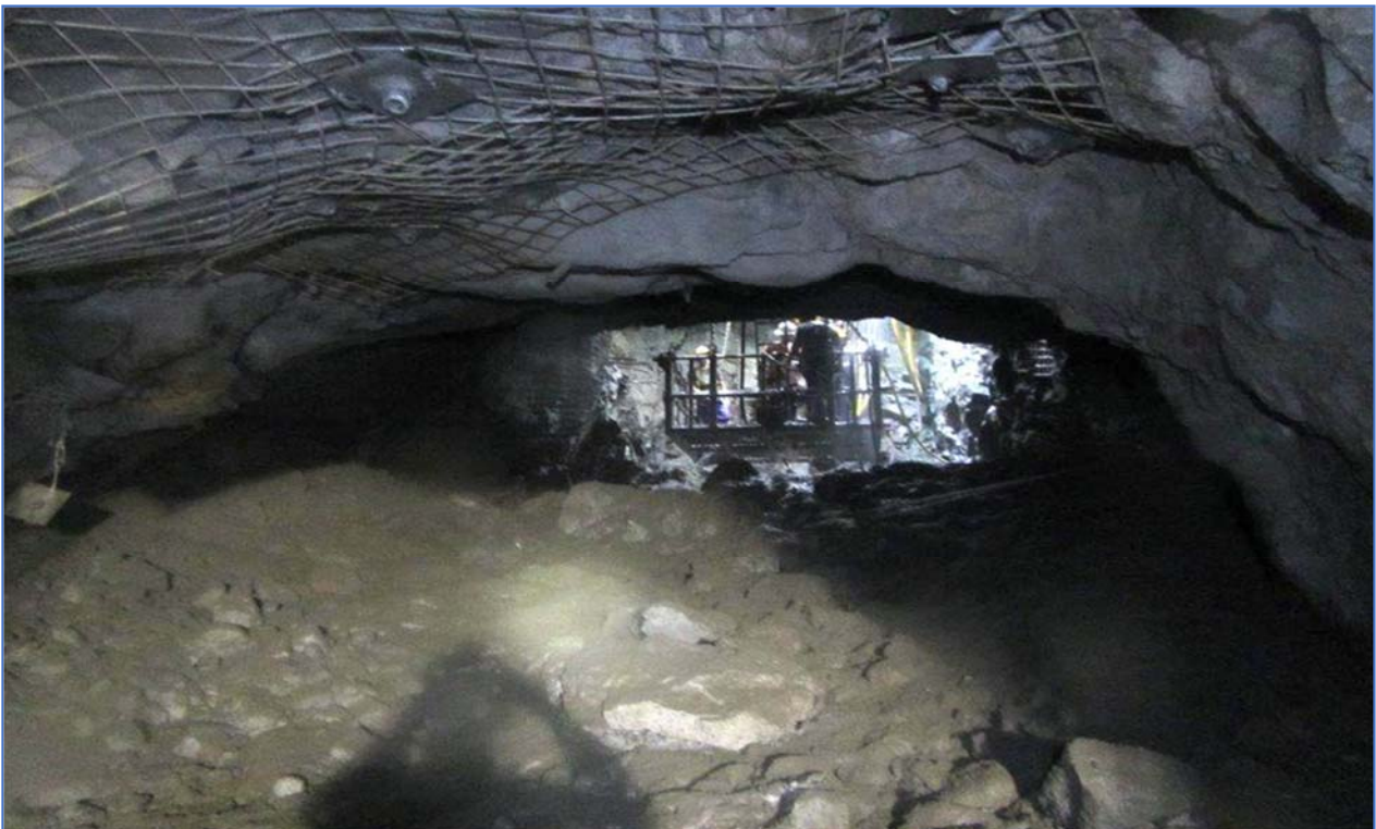
Picture 4: Shaft break through onto 5 Level
