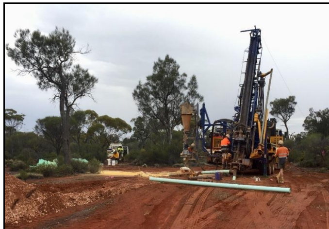
Photo 1: RC Drilling at Pinnacles Gold Project
