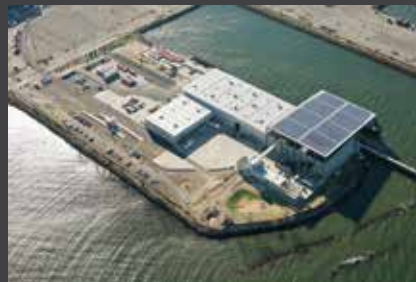
Overhead view of the MRF in Sunset Park including rooftop solar arrays and jetty.
