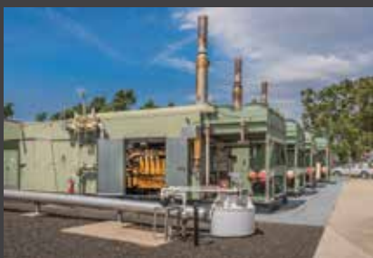
Landfill gas renewable power generation facility in Albury NSW, Australia.
