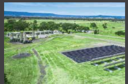
Combined solar power (foreground) and landfill gas renewable energy generation (background).
