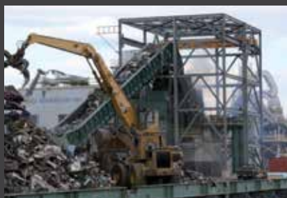
Claremont, NJ mega-shredder in operation (2006).
