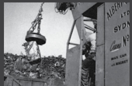
Moving baled scrap metal by magnet and crane (circa 1955).
