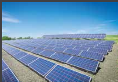
Solar generation panels in Wollert VIC, Australia.
