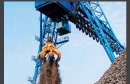
Overhead gantry crane moving material for ship loading at Newport, UK (2015).
