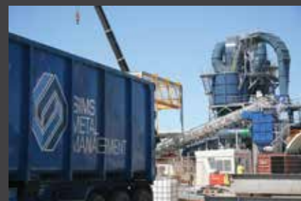
Installation of a new shredder in Kwinana WA, Australia (2016).
