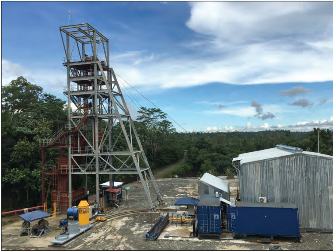
Picture 3:: E15 Head Frame and winder houses
