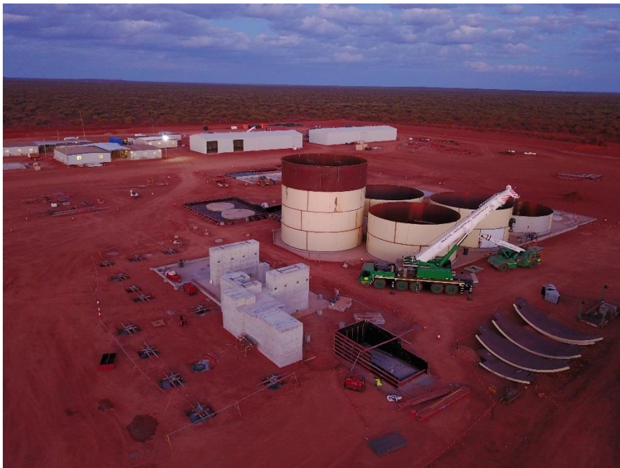
Construction of the Dalgara Gold Project Well Advanced
