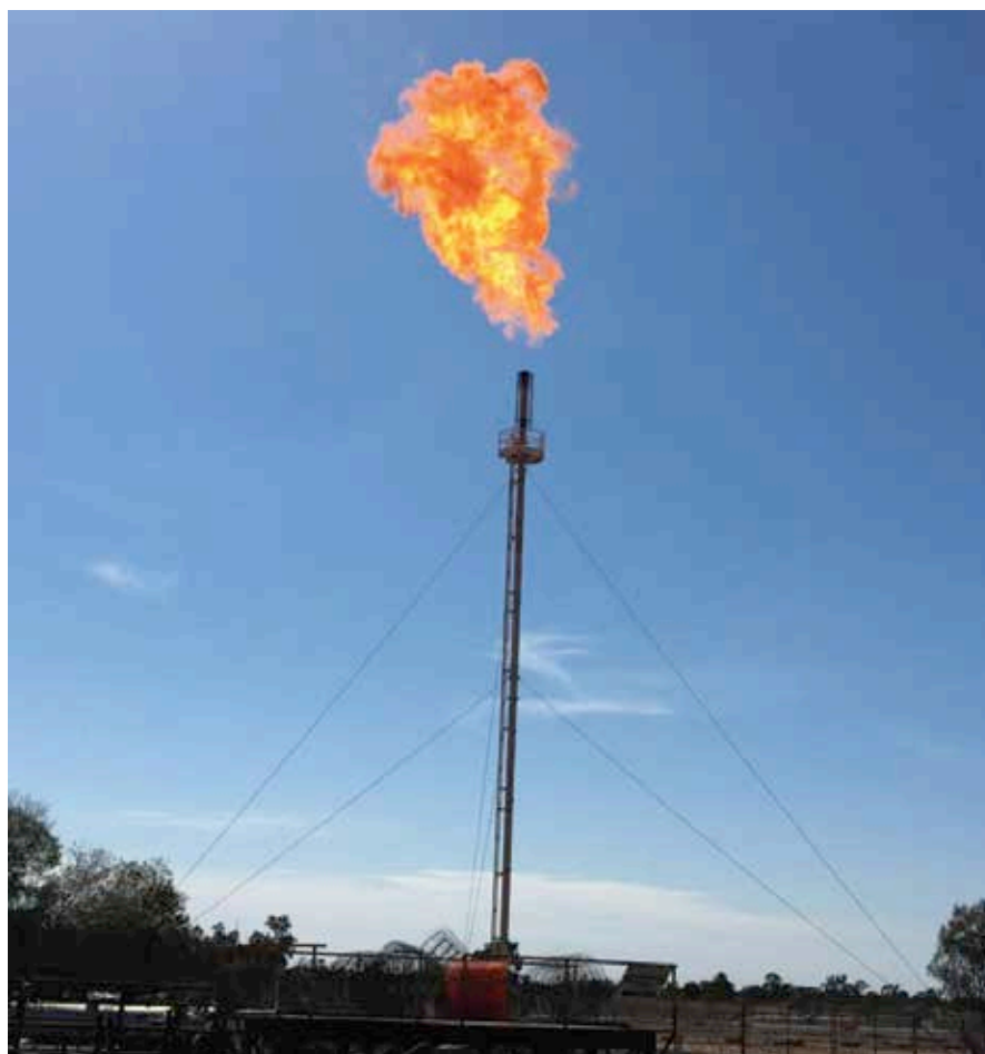
Figure 1 - Kincora Plant - flare during commissioning of dry gas circuit
