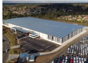
Ingleburn Distribution Centre, Sydney
