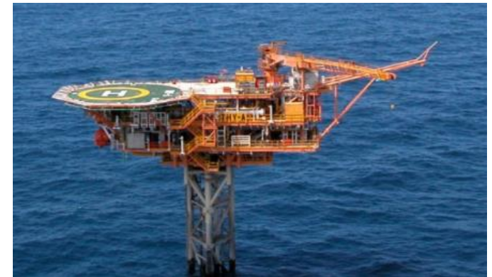
Thylacine well head platform
