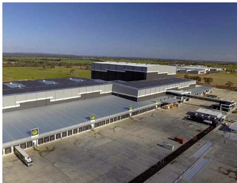
Melbourne South Regional Distribution Centre, VIC.
