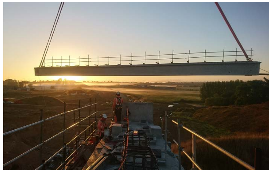
Waikato Expressway – Hamilton's City Edge
