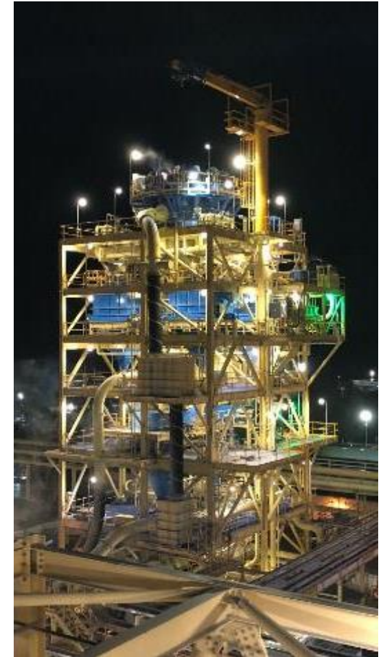
Coarse ore flotation plant, Cadia
