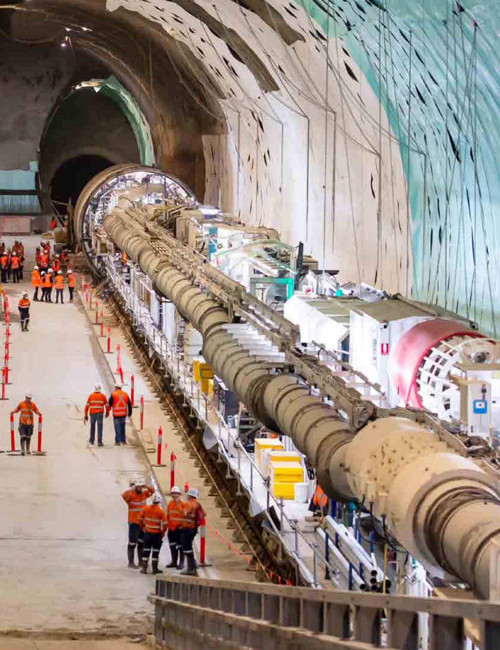
Sydney Metro City & Southwest CPB Contractors, Pacific Partnerships and UGL supported by EIC Activities, New South Wales, Australia
