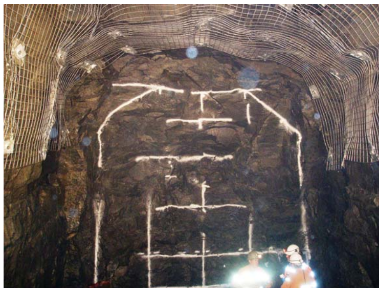
Main decline heading showing the mesh and bolt type ground support
