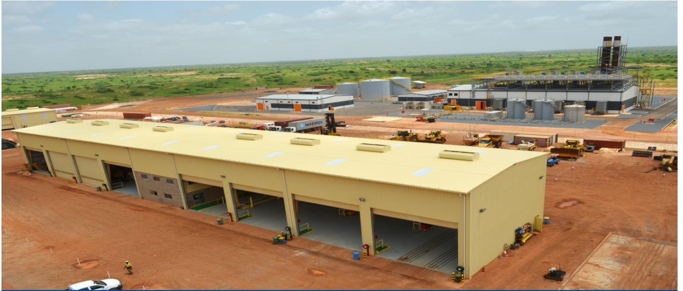
Power Station in background and Workshop in foreground
