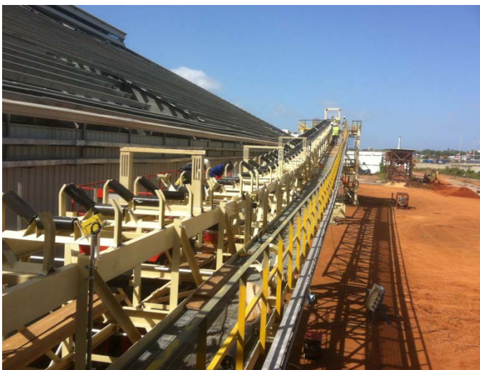
Part of port conveyor system
