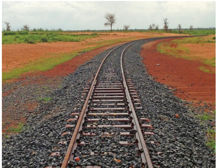
New rail spur
