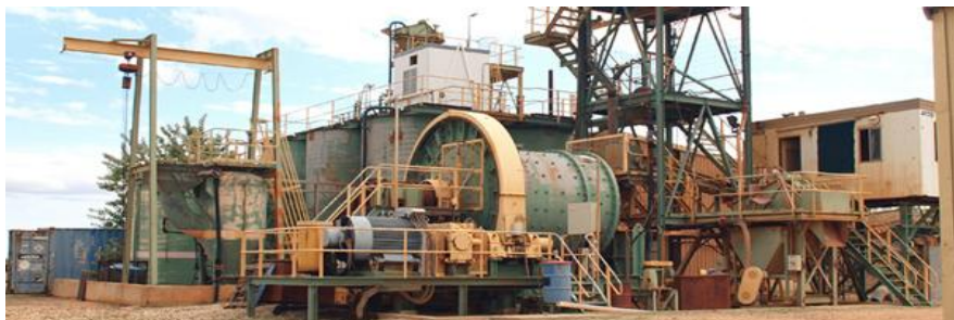
Existing Processing Plant at Nicolsons
