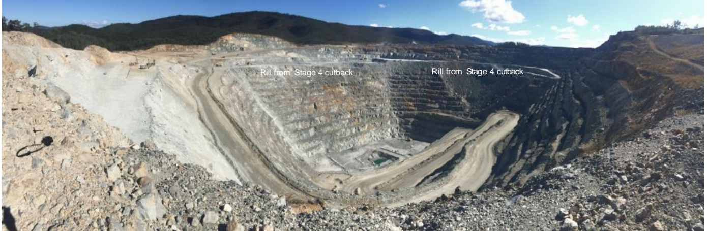
Mt Rawdon open pit July 2015 looking north to stage 4 cutback – north and west walls currently being stripped
