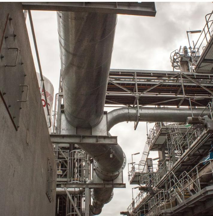
*Ducting for odorous air extraction, entering biofilter odour management system.*
