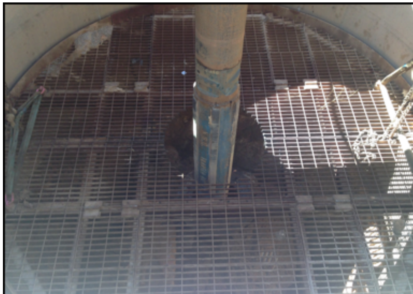
3 m diameter ventilation raisebore broken through to surface
