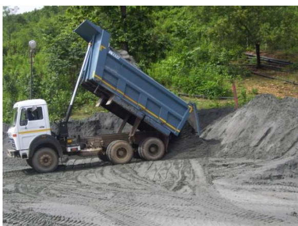
Shaft 3: Tailings backfill operation
