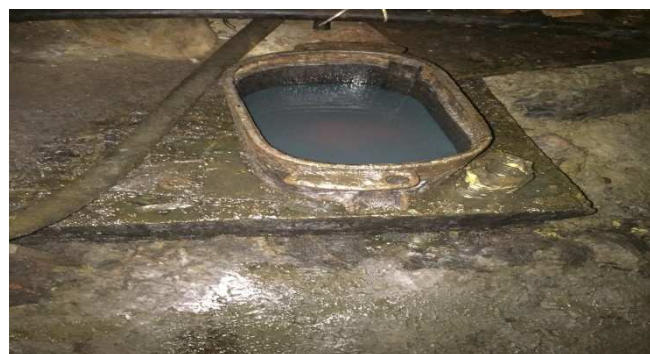
Shaft 3: Used Oil collection in underground Pump chamber
