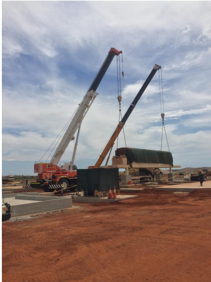
Kiln being installed
