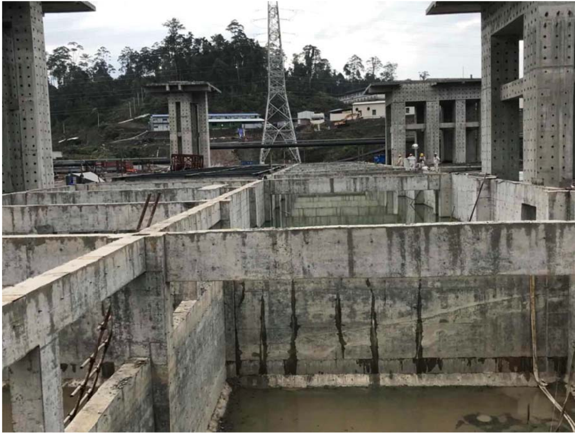
Foundation for Ranger Nickel slag pool
