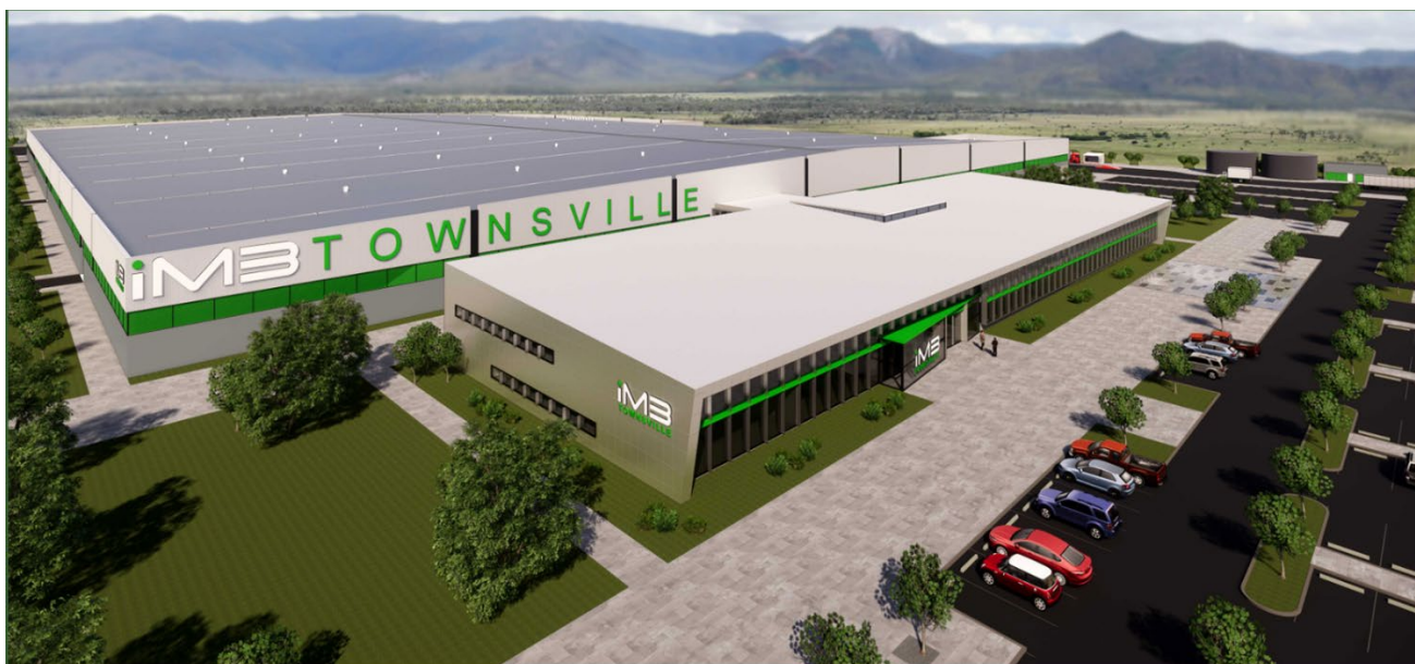
Figure 1: GHD developed LIB Manufacturing Plant Aerial View
