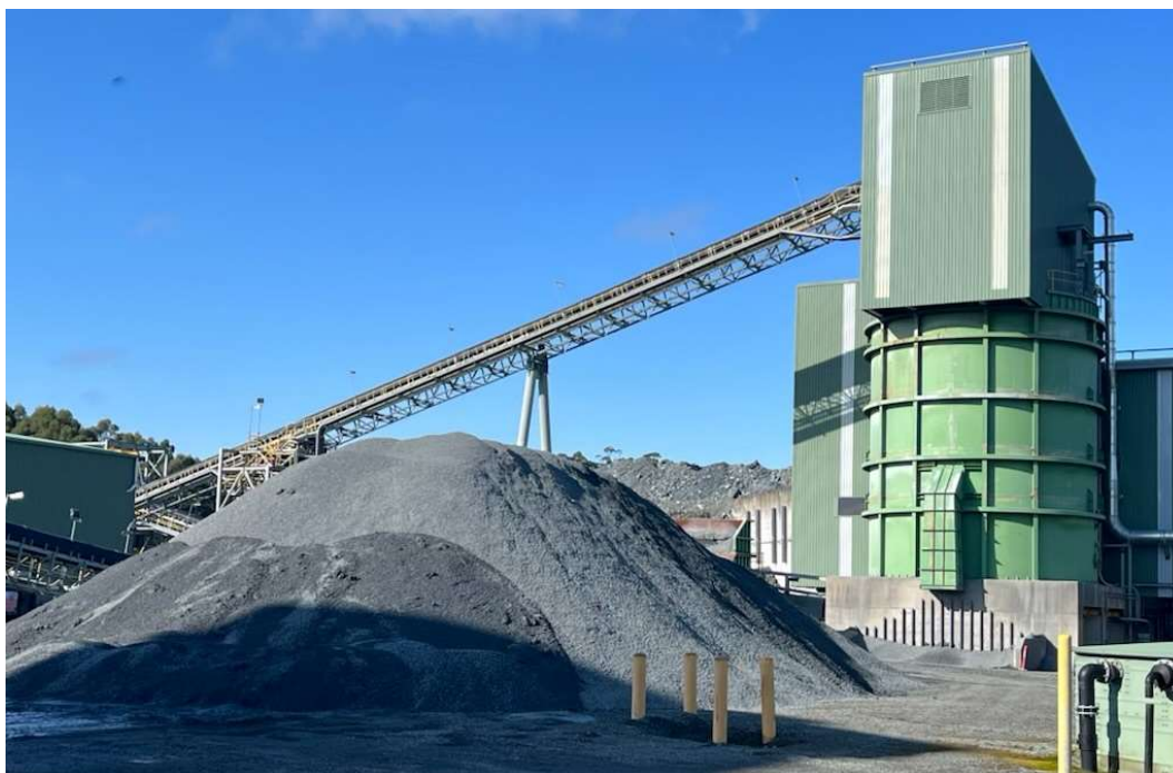
Fine Ore overflow stockpile, with fine ore bin and crusher house behind
