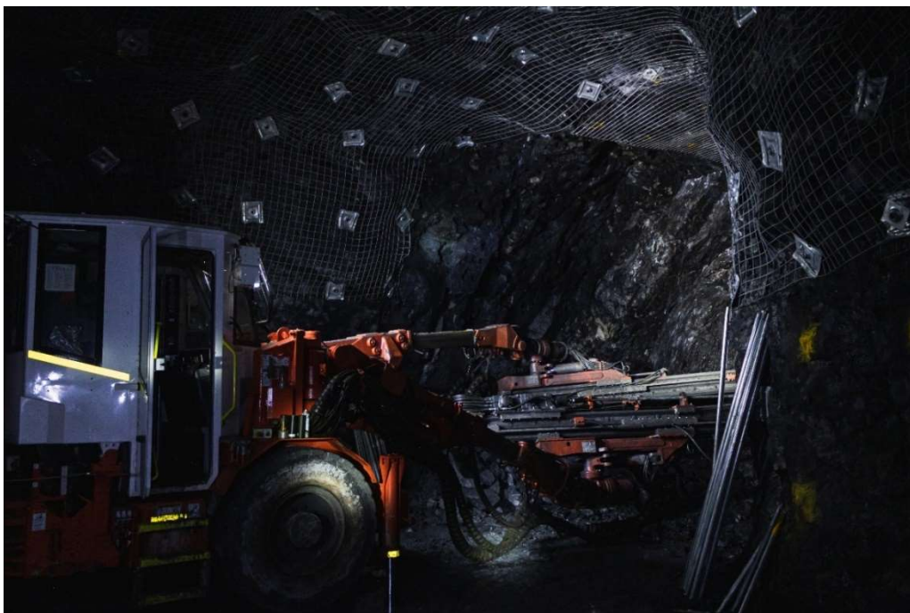
Jumbo installing ground support underground at Avebury
