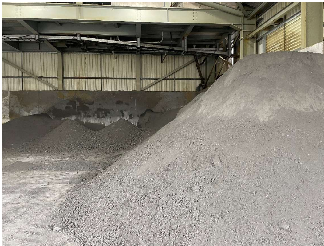
Finished concentrate in the concentrate storage bay on site at Avebury, ready for transport to port
