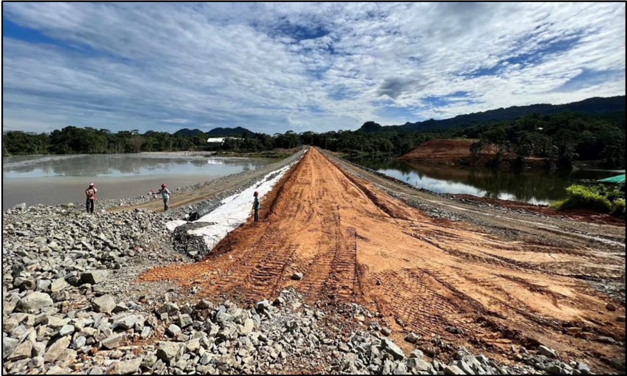
Photo 1. Ongoing construction extension of TSF#5B. Crest view.
