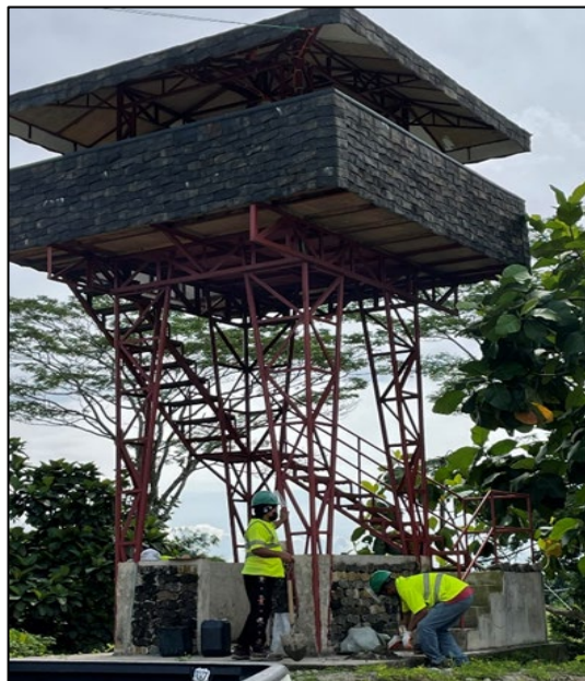
Photo 31. Upcycling of safety boots and used HDPE pipes as roofing and walling of view.
