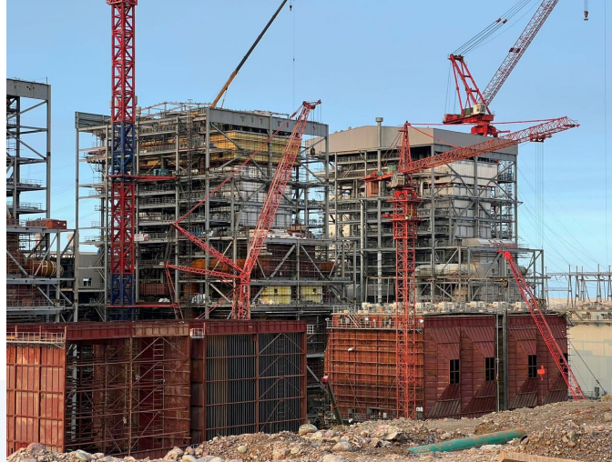
Construction progress at the ONI power plant
