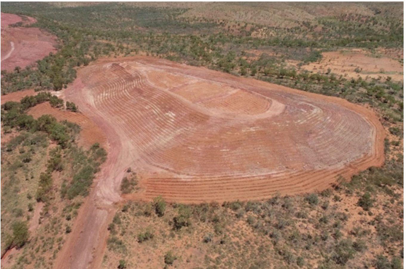
Figure 4: Profiling, topsoil spread, drainage and cross-rip completed.
