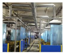
Newly installed weld fume and dust extraction system at an APG supplier
