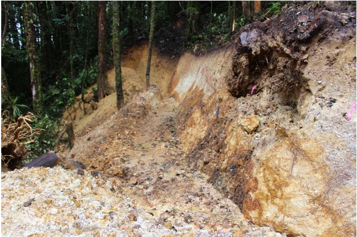
Figure 20. A trench exposure at Mt Wipi showing variable alteration, weathering and iron staining.
