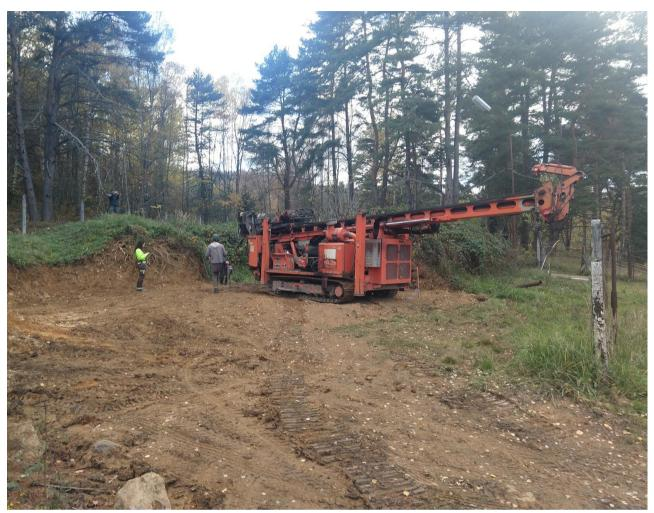
**Figure 16:** Diamond drill rig set up at the first target area, site preparation completed, location of drill hole SSD-01
