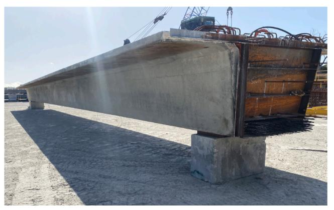
First beam cast in new multipurpose, high-capacity adjustable stressing bed – Bennett Brook Bridge
