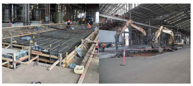
Figure: Filtration Area Formwork (left) and Filtration Area Excavation (right)
