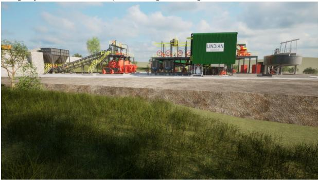
Image 7: Preliminary schematic of plant design from ground level. Existing retaining wall (left), ball mills (centre left), recovery circuit (centre) and tailings thickener (right)
