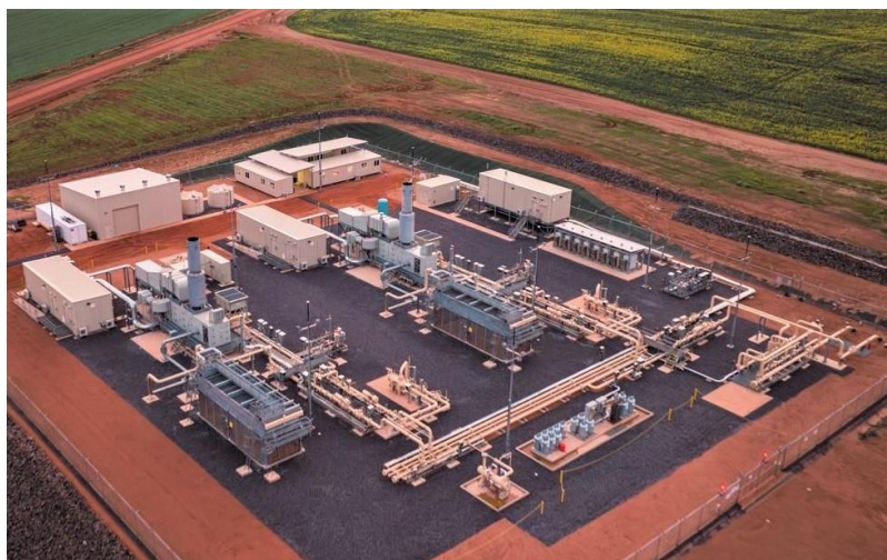
APA Ambania Compressor Station – Completed 2023
