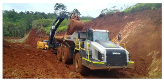
Removal of overburden in the first ore blocks for the mining of ore planned to commence in October 2023
