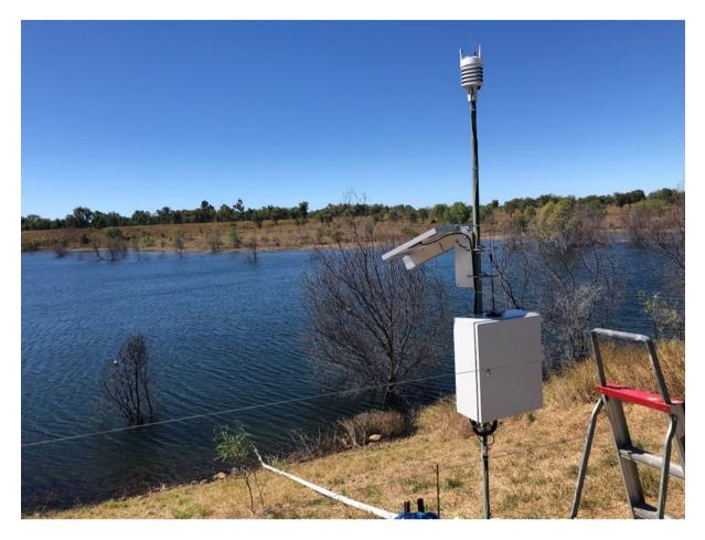
Figure 34: New Weather Station to Assist in Environmental Monitoring Installed at Yandan.
