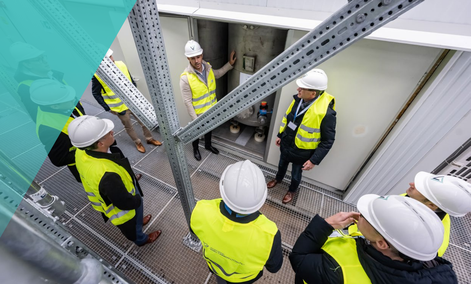
FIGURE 3 IN-HOUSE DESIGNED LITHIUM EXTRACTION OPTIMISATION PLANT
