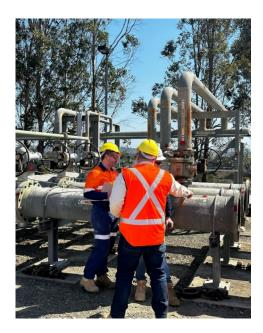
Part of the newly acquired RPGP - Gas will be delivered to the Carpentaria Gas Plant via the buried gas gathering system at low pressures to maximise well deliverability
