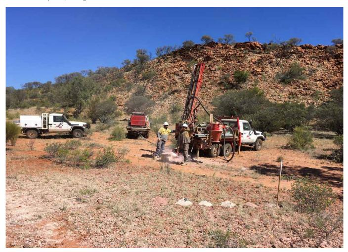
Figure 4: Aircore drilling at the Dingos Rest South prospect August 2023
