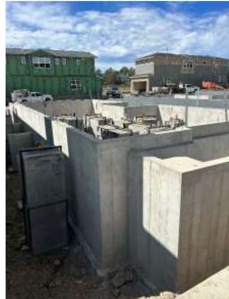
Figures 1 & 2 First EdenCrete® Pz7 project- Foundation walls for home development – Colorado
