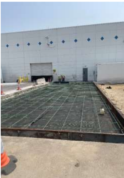
Figures 5 &6 DIA- United Airlines Cargo Area – concrete panel replacement.
