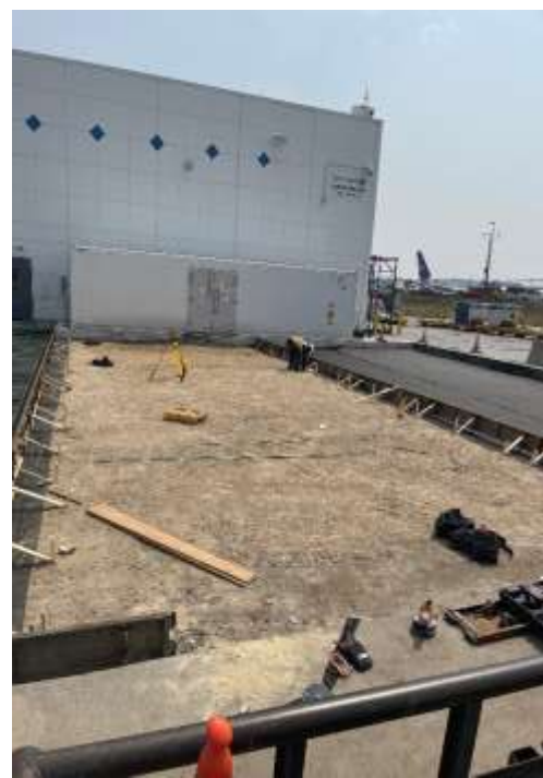
Figures 5 &6 DIA- United Airlines Cargo Area – concrete panel replacement.
