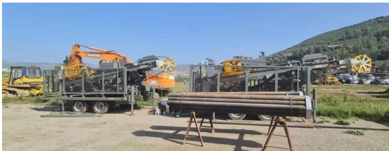
Figure 1 - Geotechnical drilling equipment at Tala Hamza
