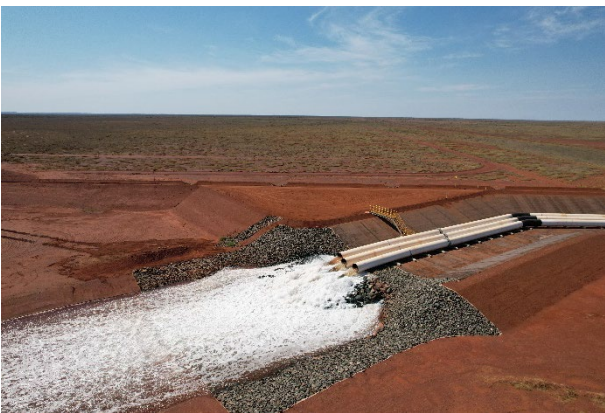
Figure 3: Commissioning of transfer station 2/3
