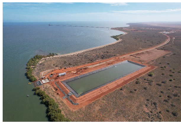
Figure 4: Construction of the secondary seawater intake station
