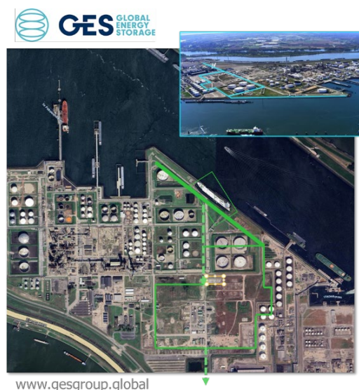
GES Terminal Site at the Port of Rotterdam, Netherlands
